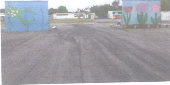
East side of Wall nos. 1 & 2
