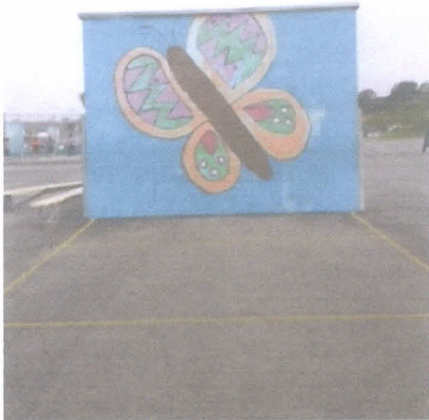
South side of Wall no. 3
