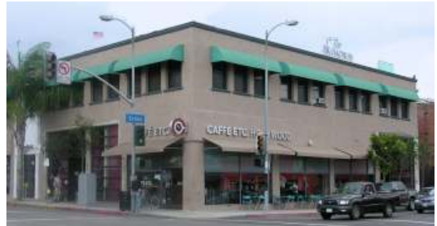
Standard 3a Example. Buildings occupying corner lots can create a welcoming pedestrian environment by articulating the ground-floor facades along both Lincoln and the intersecting street.
