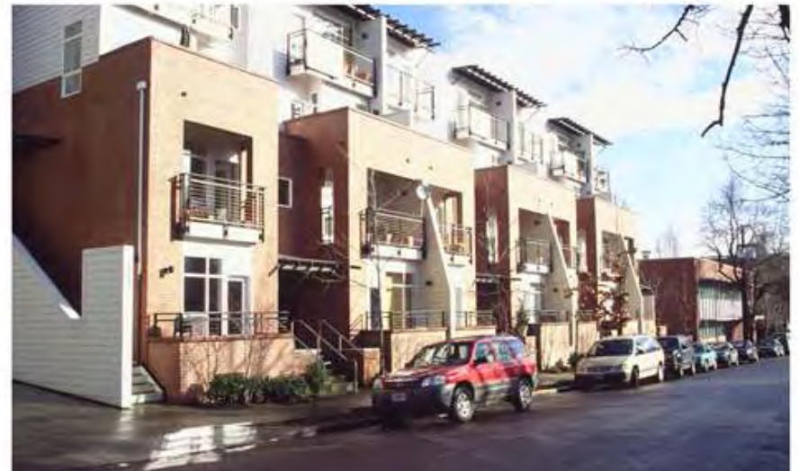
Standard 1d Example. For portions of projects where the ground floor contains residential units, individual entrances to the ground-floor units are encouraged. Entrances should be slightly set back from the property line and elevated two to five feet.
