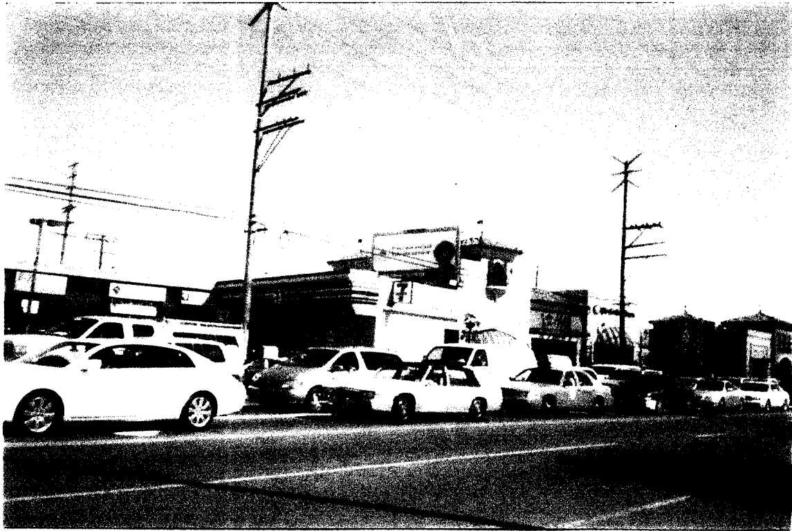
15. View of commercial uses easterly of site
