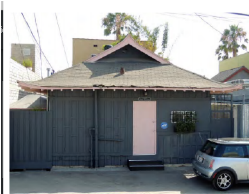
Address: 1641 S. Abbot Kinney Boulevard Name: Pacific Electric Venice Short Line Ticket Building Date: 1911
