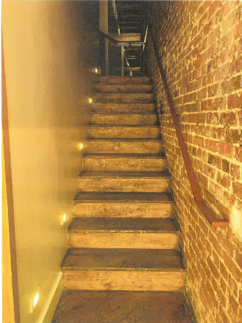
Stairs between the first floor and the mezzanine level
