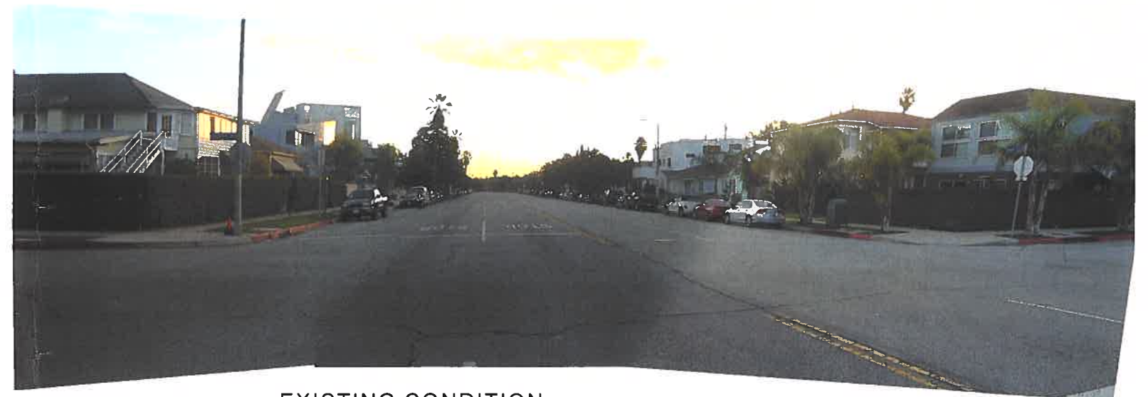
EXISTING CONDITION GRAND BLVD. AT ANDALUSIA AVE. FACING EAST
