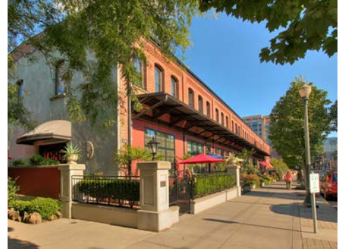
Awnings, umbrellas, and enclosures break down a long building frontage and help create a human-scaled frontage at the sidewalk in Portland, Oregon.
