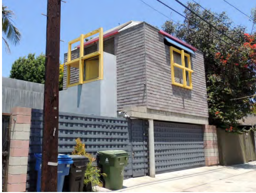
Address: 932 W. Amoroso Place Name: 2-4-6-8 House Architects: Thom Mayne and Michael Rotondi Date: 1979
