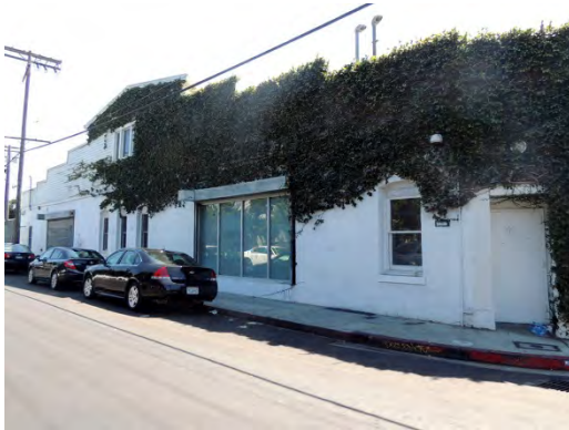
Address: 200 E. Mildred Avenue Name: Venice Gondola Building Date: 1913
