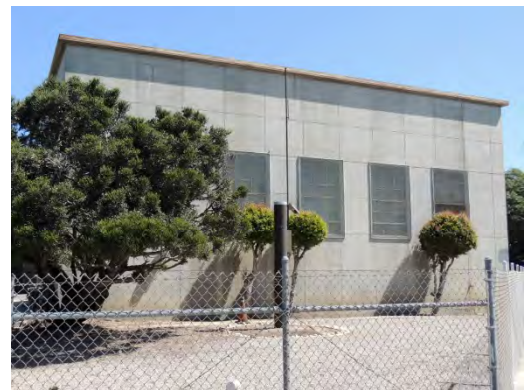
Address: 314 E. Brooks Avenue Name: Electric Avenue Pump Plant Date: circa 1950
