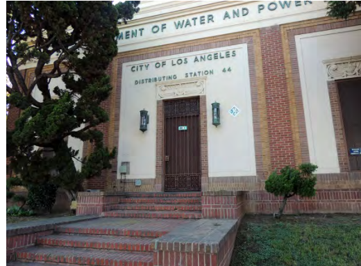
Address: 911 S. Lincoln Boulevard Name: L.A. Department of Water and Power Distributing Station No. 44 Date: 1928
