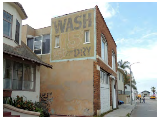
Address: 26 E. Brooks Avenue Name: Wash/Dry Wall Sign Date: Unknown
