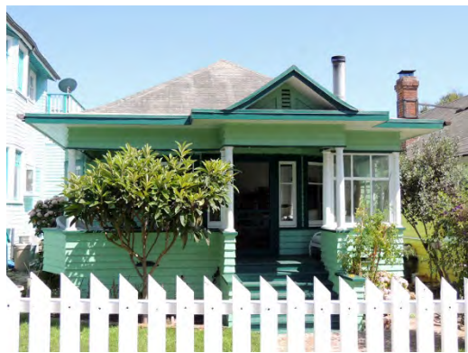
Address: 26 E. Thornton Avenue Date: 1902
