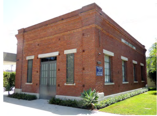
Address: 660 E. Venice Boulevard Name: Southern California Edison Substation Date: 1923
