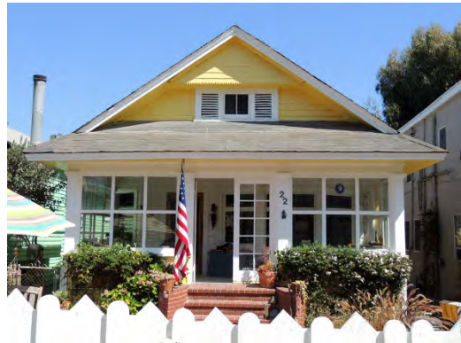
Address: 22 E. Thornton Avenue Date: 1905
