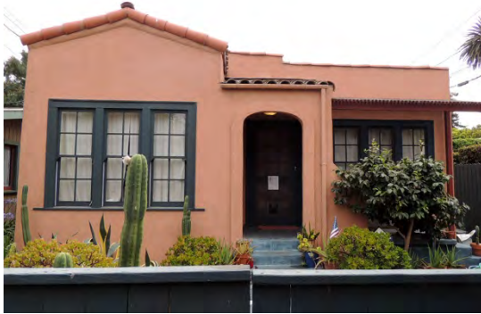
Address: 1615 S. Shell Avenue Date: 1925
