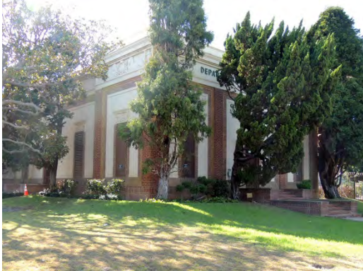
Address: 911 S. Lincoln Boulevard Name: L.A. Department of Water and Power Distributing Station No. 44 Date: 1928
